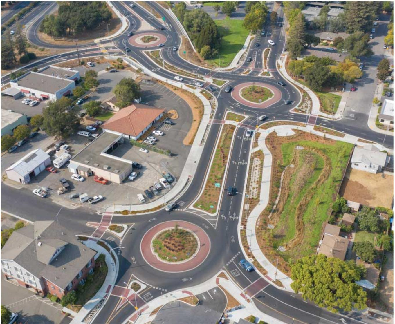
THE CALIFORNIA BLVD AND 1ST/2ND STREETS ROUNDABOUT PROJECT IN NAPA, CALIFORNIA, WAS DESIGNED TO RELIEVE TRAFFIC CONGESTION, IMPROVE TRAFFIC SAFETY AND TRAFFIC OPERATIONS, AND MINIMIZE QUEUES AND DELAY FOR ALL THREE INTERSECTIONS.
